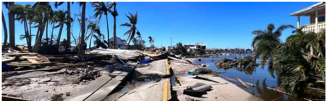
Top left: FWC Hurricane Ian responder; top right: Hurricane Ian damage to a SW FL neighborhood; bottom: Hurricane Ian road damage
